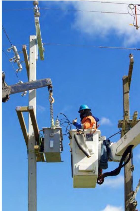
Photo 9 Pole Mount Transformer installation 2012
