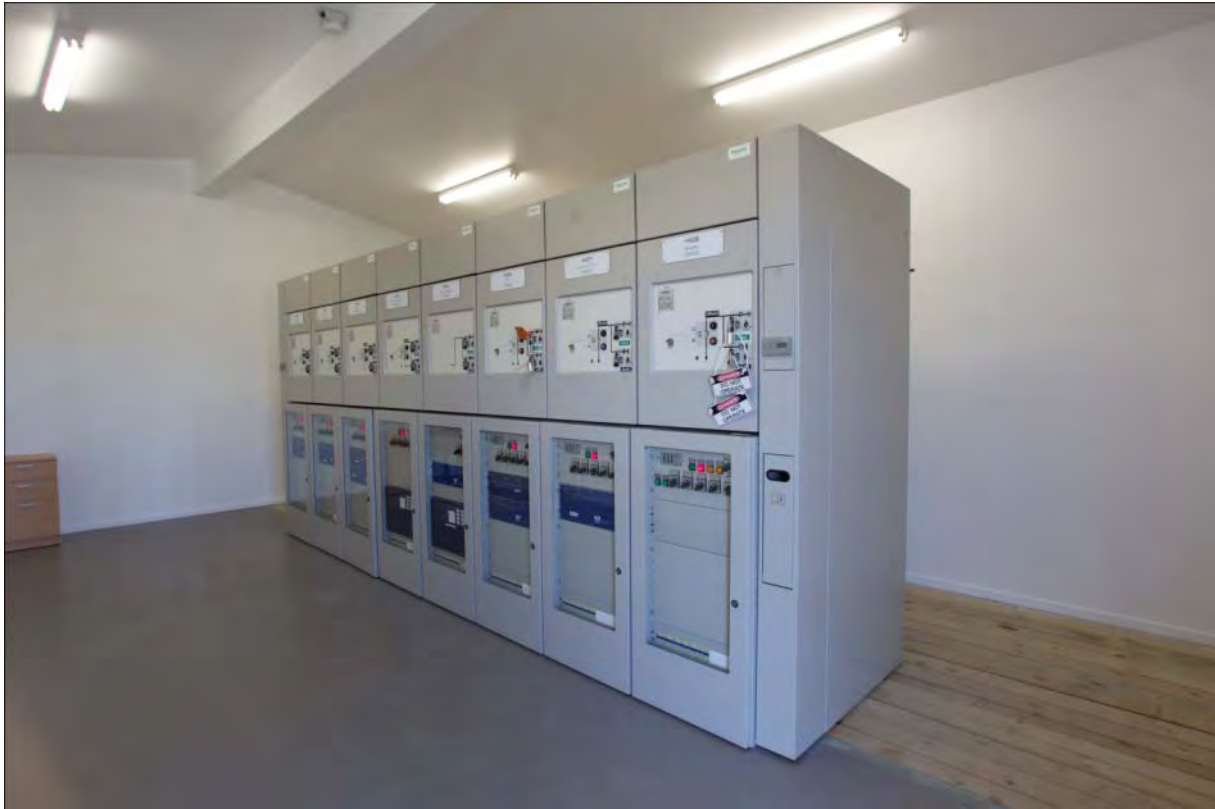
Photo 6 New 33kV indoor switchgear at Te Kauwhata Substation
