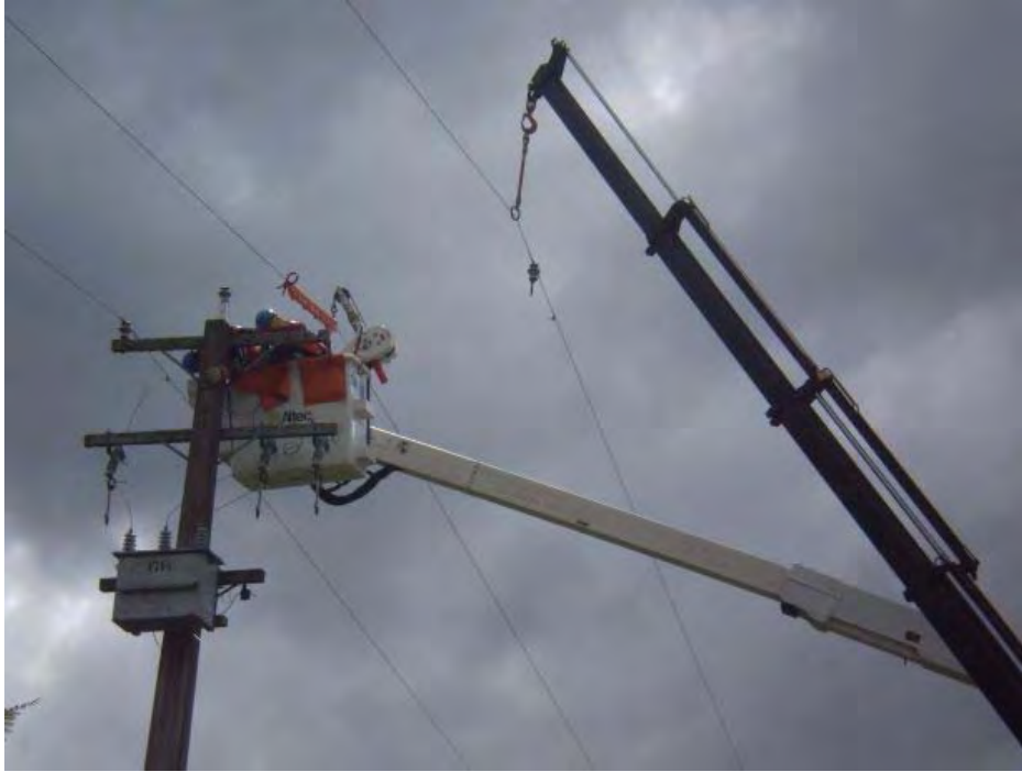
Photo 23 Live Line Installation of Delta Support
