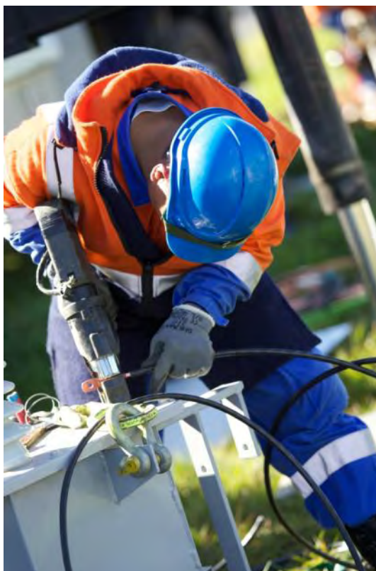
Photo 5 Preparing a pole mount transformer for installation
