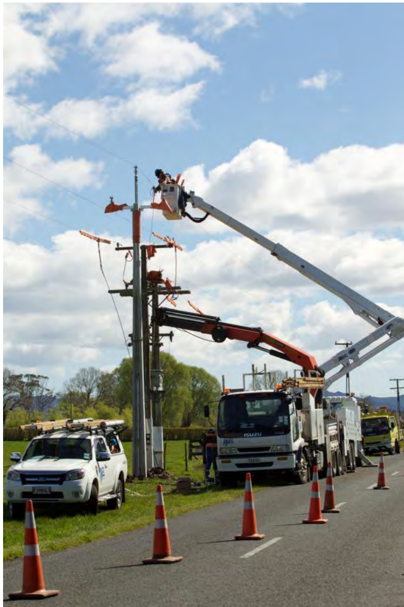
Photo 2 Live Line Pole replacement 2012
