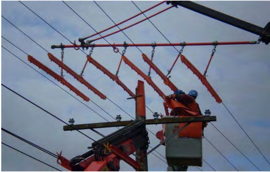
Photo 18 Live Line Replacement of HV Insulators 2012
