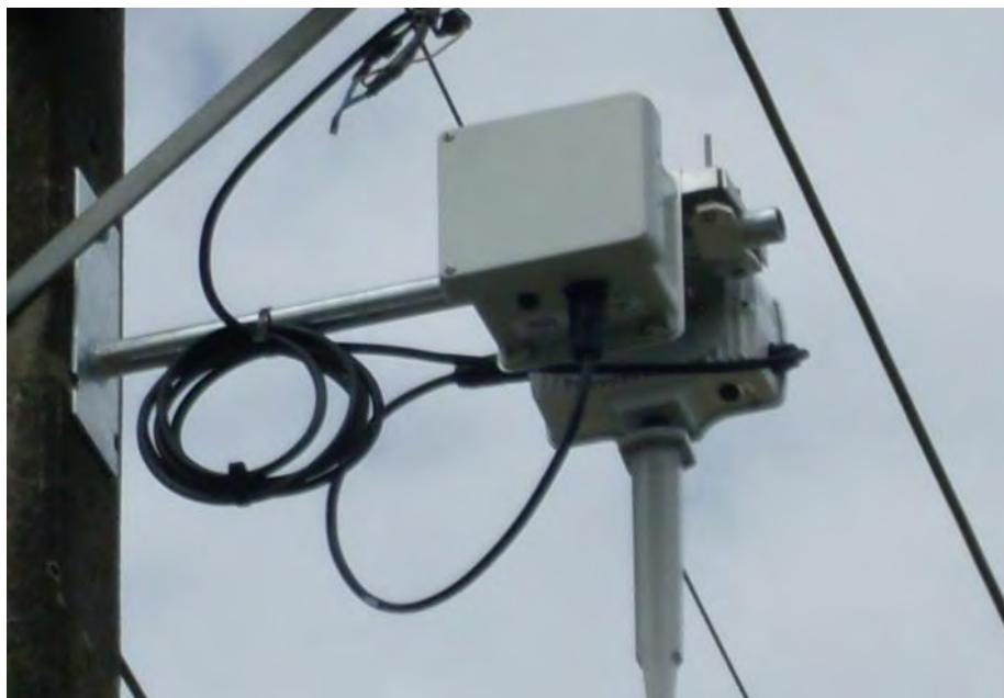
Photo 20 RF Mesh relay installed on a Pole
