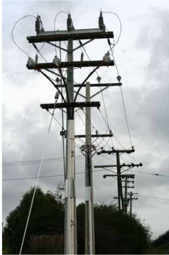
Photo 3 33kV and 11kV line termination poles
