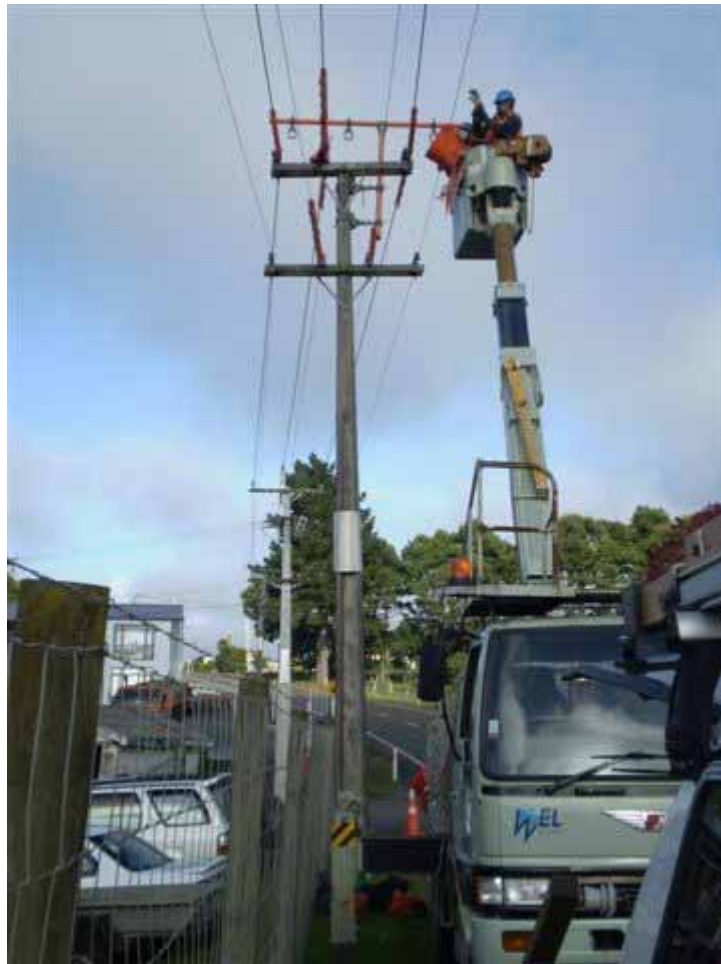
Photo 13 Live Line Crossarm Replacement
