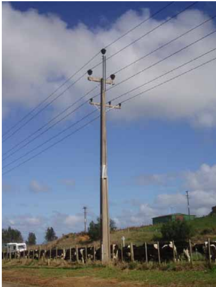
Photo 8 33kV – 11kV Standard Configuration
