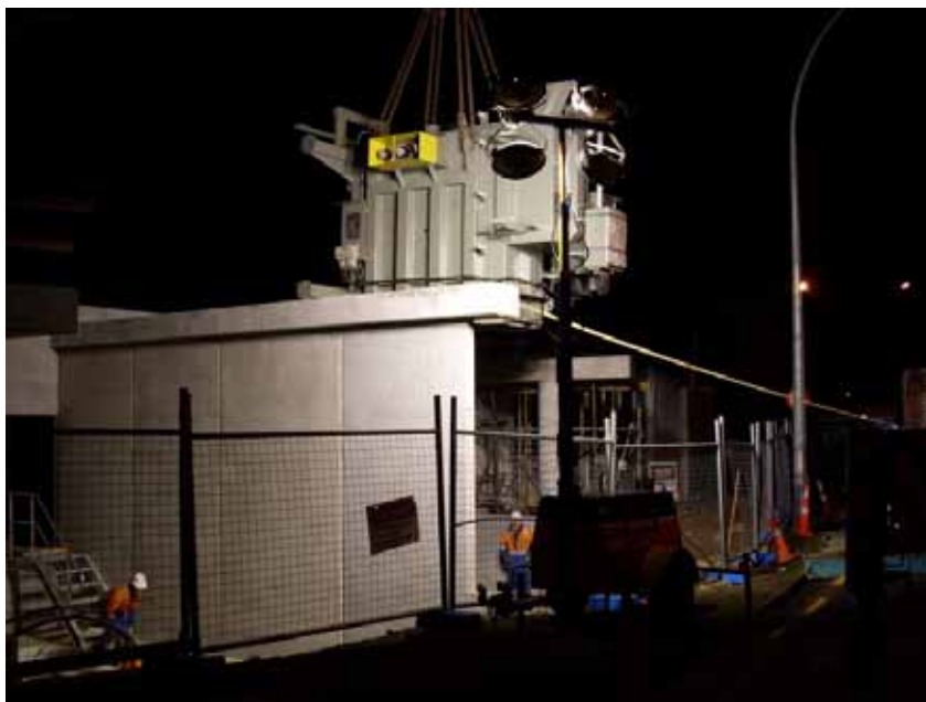
Photo 14 Transformer installation at the Cobham Drive zone substation
