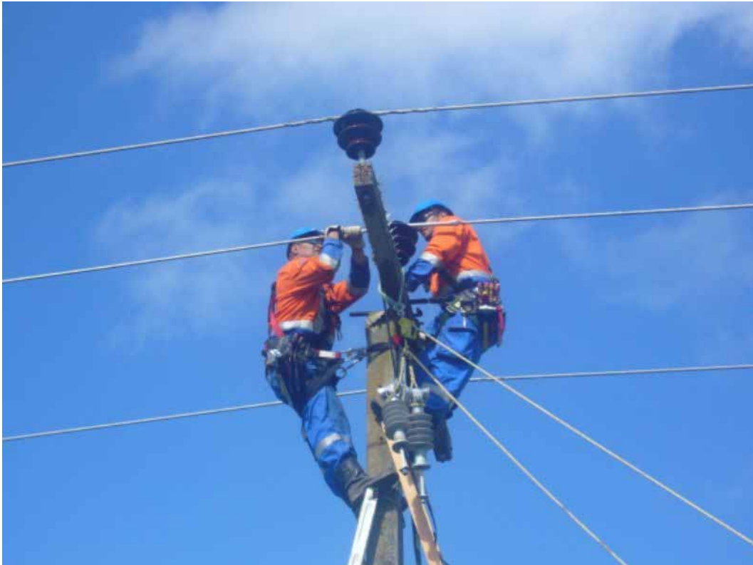
Photo 4 33kV Insulator Replacement
