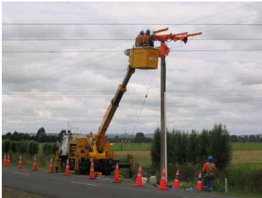
Photo 10 Live Line Maintenance
