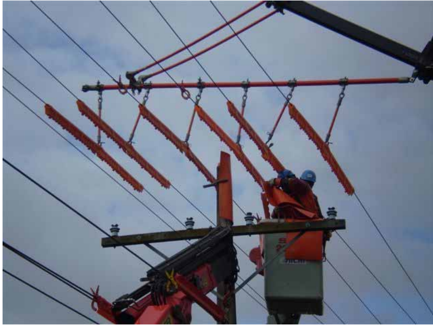
Photo 18 Live Line Replacement of HV Insulators
