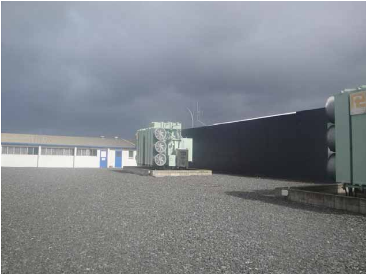
Photo 1 33/11kV transformers and building at Avalon Drive substation
