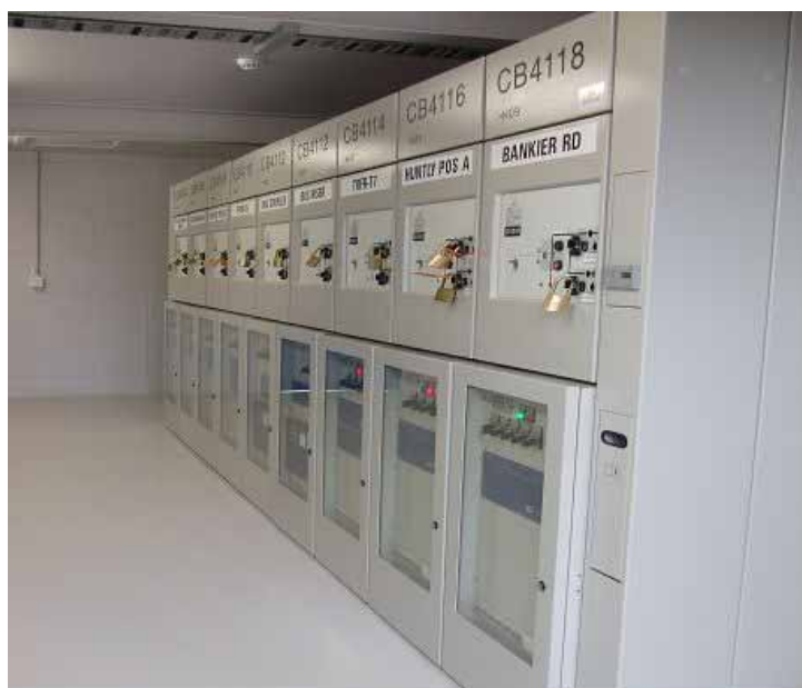
Photo 20 33kV Indoor gas-insulated switchboard
