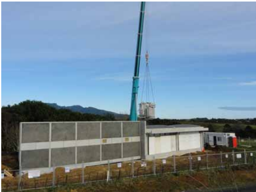
Photo 25 Transformer being installed at the new Raglan Substation
