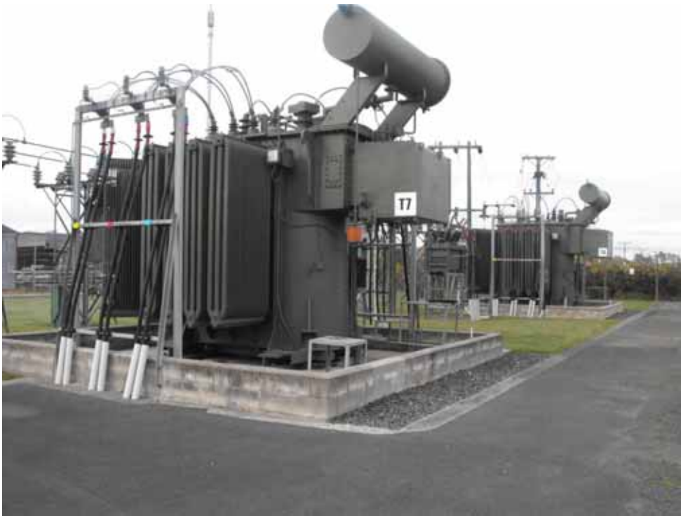
Photo 16 33/11kV transformers at Latham Court Substation
