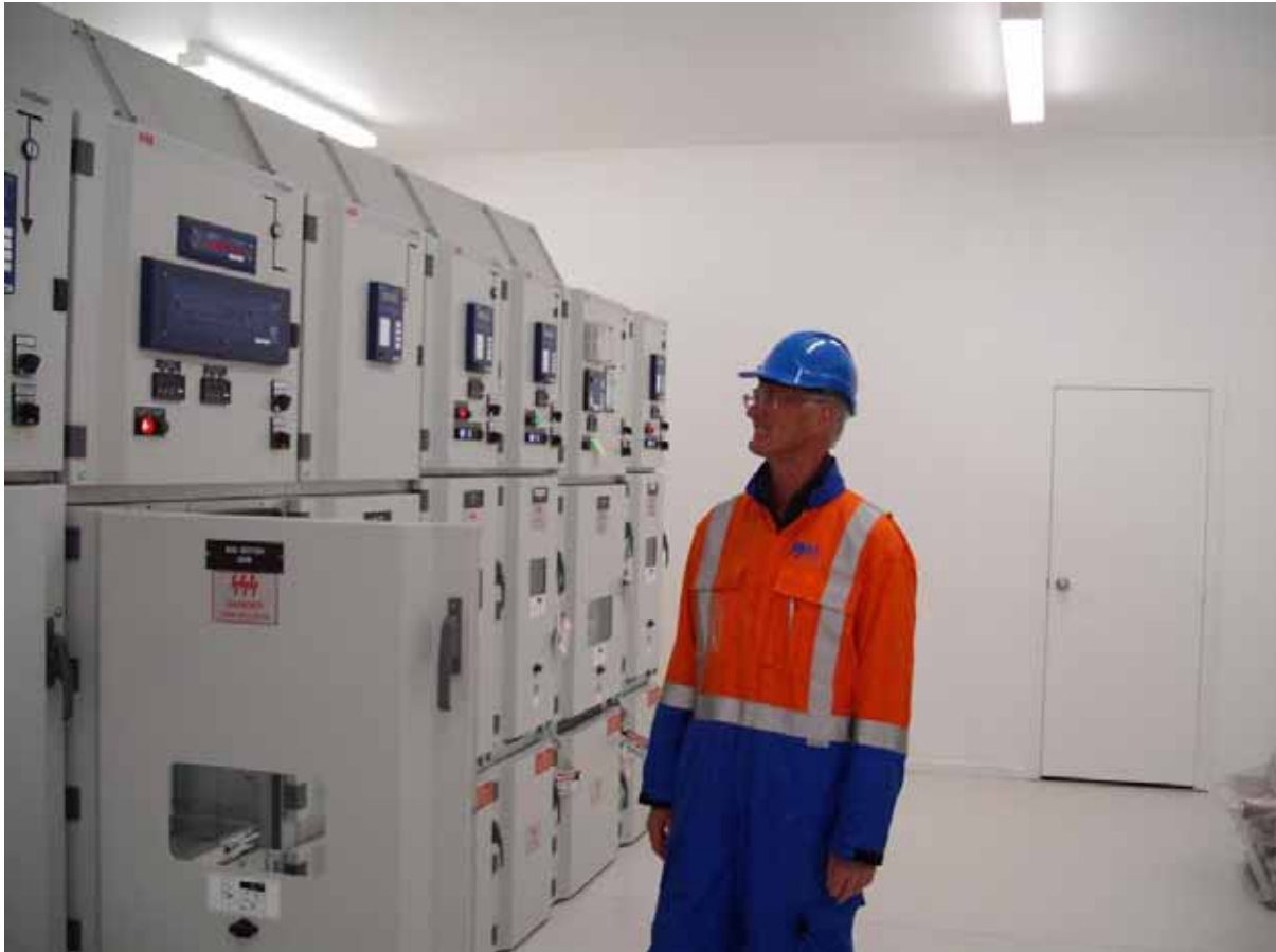
Photo 22 Inspection of the 11kV switchgear at Whatawhata substation
