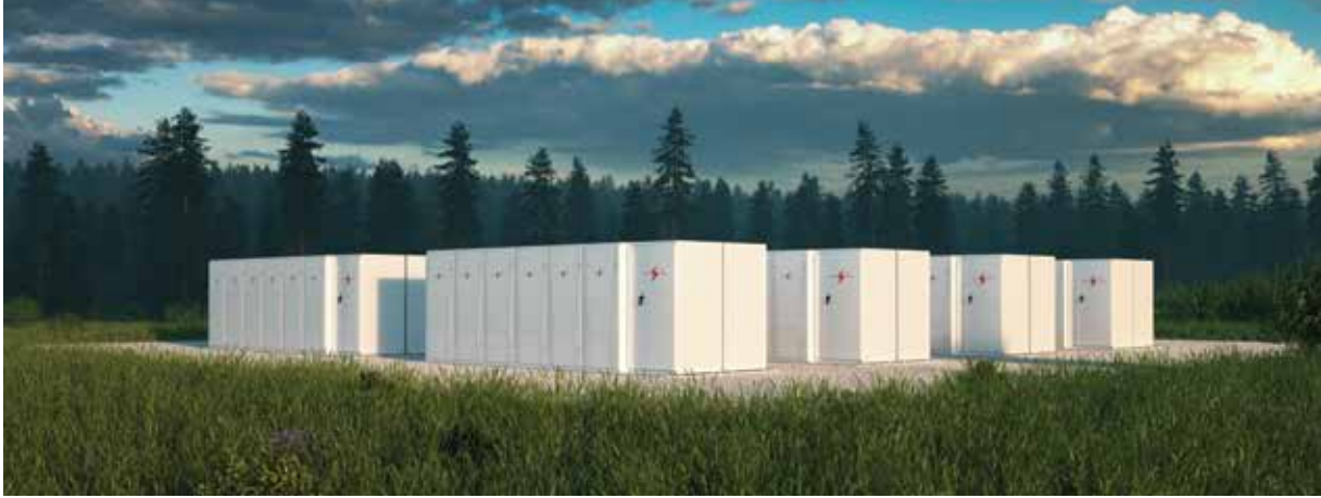
An example of a Battery Energy Storage System (BESS).
