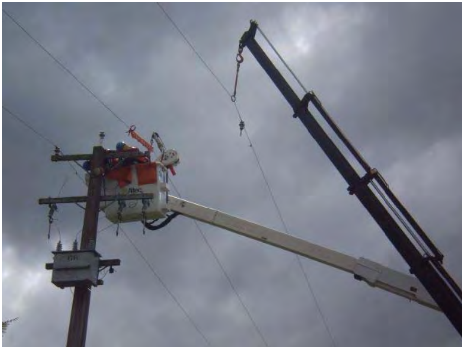
Photo 24 Live Line Installation of Delta Support
