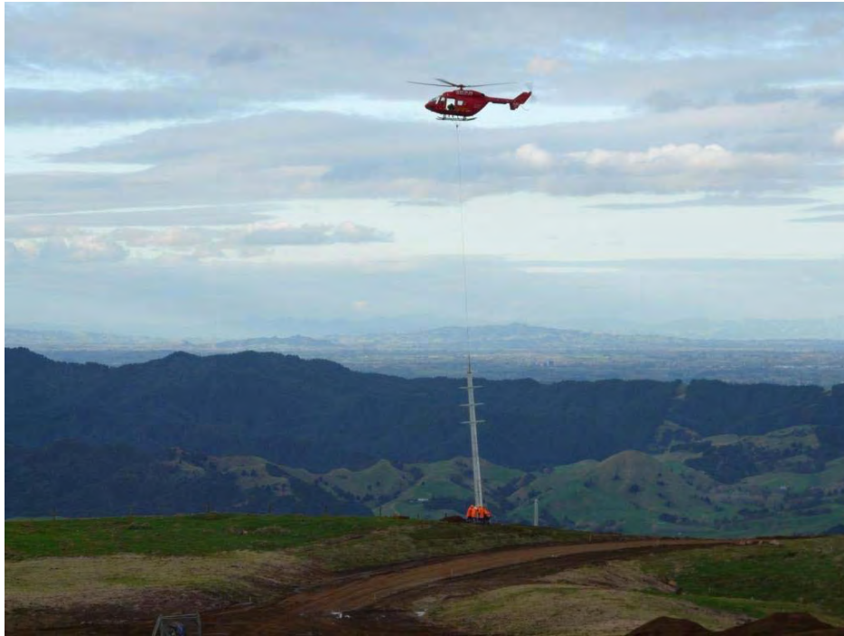
Photo 17 Construction of the 33kV transmission line
