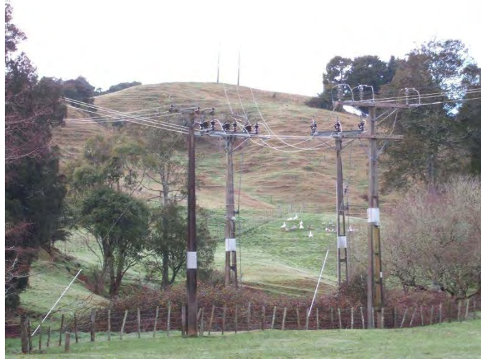
Photo 16 33kV Air Break Switches
