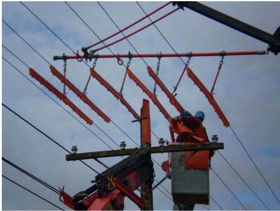
Photo 18 Live Line Replacement of HV Insulators
