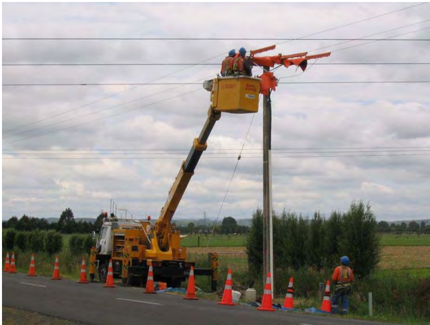
Photo 10 Live Line Maintenance
