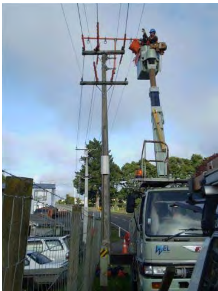
Photo 13 Live Line Crossarm Replacement
