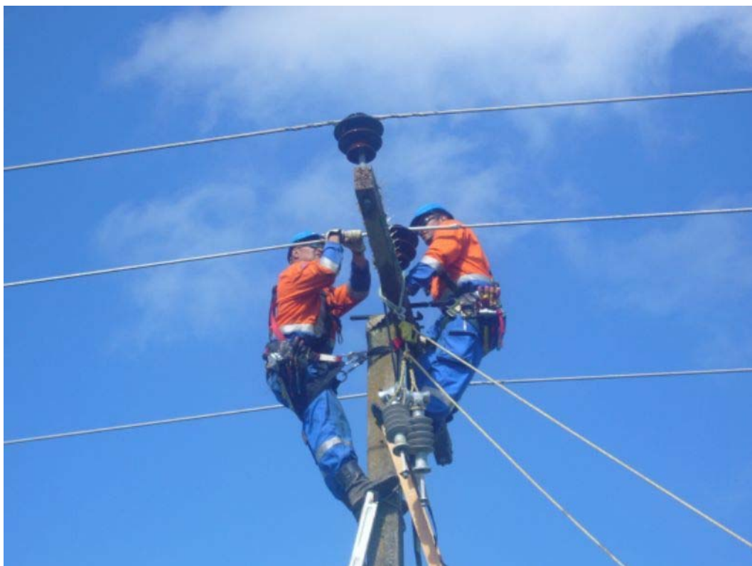
Photo 5 33kV Insulator Replacement
