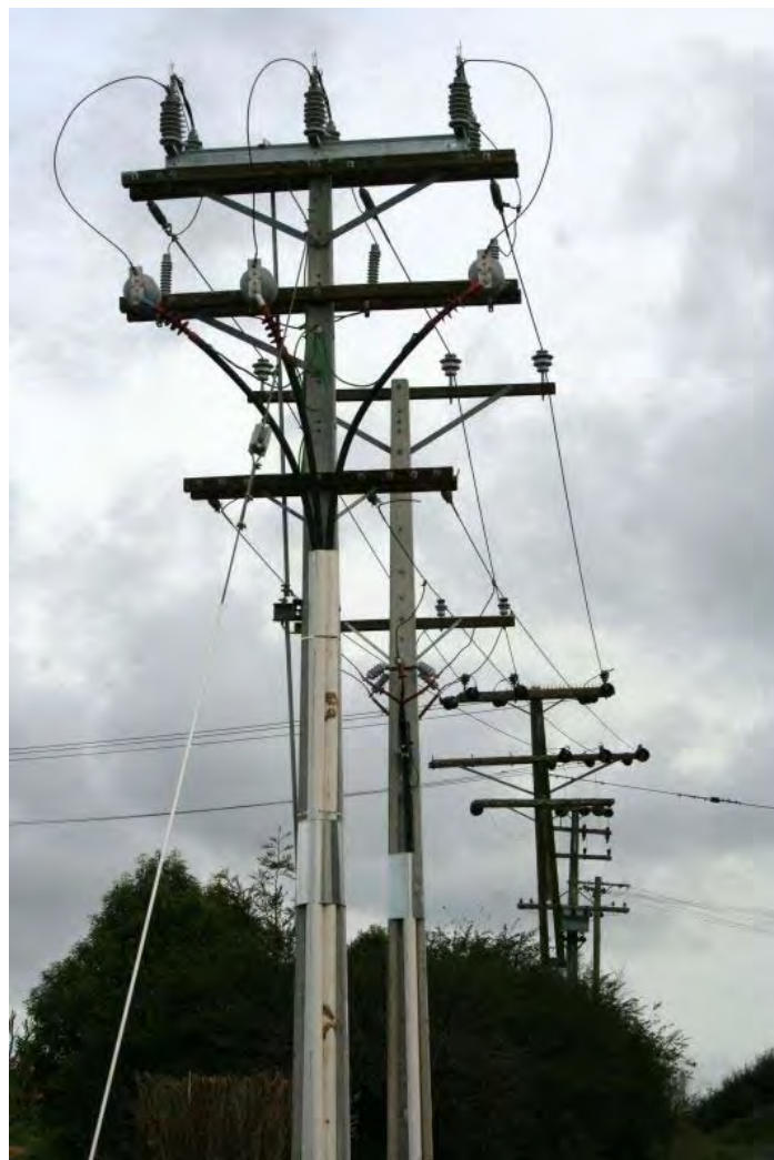
Photo 4 33kV and 11kV line termination poles
