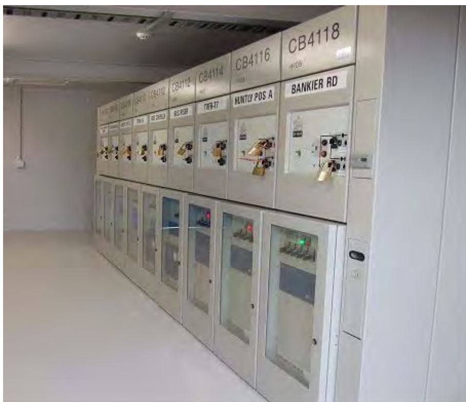
Photo 20 11kV Indoor gas-insulated switchboard
