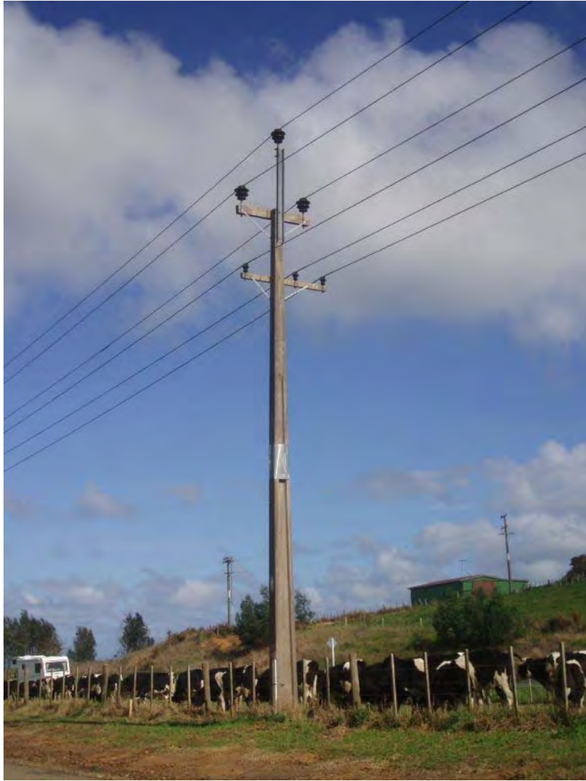
Photo 8 33kV – 11kV Standard Configuration
